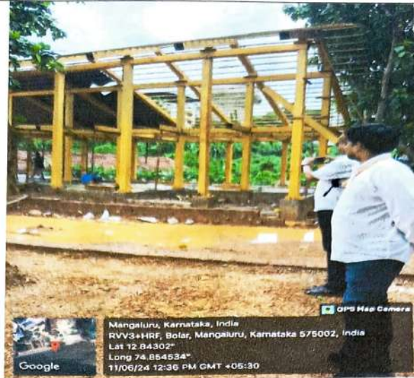
Temporary shed on concrete footing to facilitate river view
