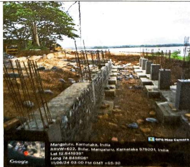
Construction of concrete footing
